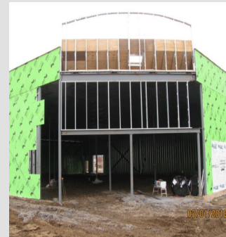
The store's future entrance
