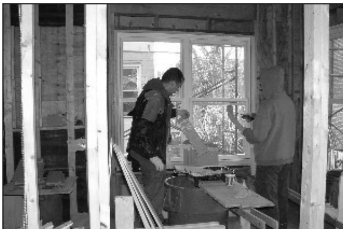
Workers continue renovation work at Westhab's project in Yonkers.
