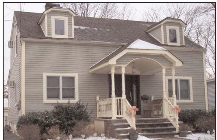
The New Jersey-based nonprofit, Homefirst, purchased this two-family home (pictured below) to create permanent supportive rental housing for disabled and homeless individuals and families living in Union County.
